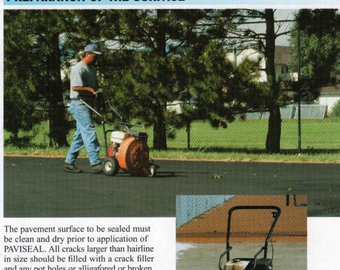
and any pot holes or alligatored or broken up pavement should be repaired prior to application of PAVISEAL.
